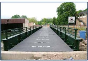
Modular Drive Through Bridge construction for a miniature railway at Wicksteed Park in Kettering, Northamptonshire. 27.3m long by 3.75m internal width, installed in June 2014.
