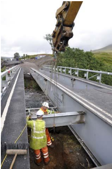
A82 Bridge of Orchy
