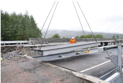
A82 Bridge of Orchy
