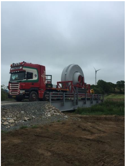
Minnygap Wind Farm, Moffat
