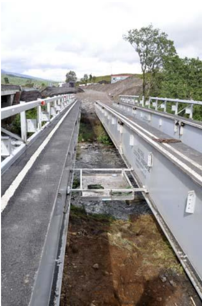
A82 Bridge of Orchy
